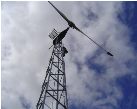
Figure 3.4: Deployed Tip-Brake
