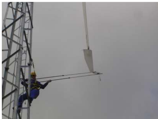
Figure 3.5: Re-setting Tip-Brakes
