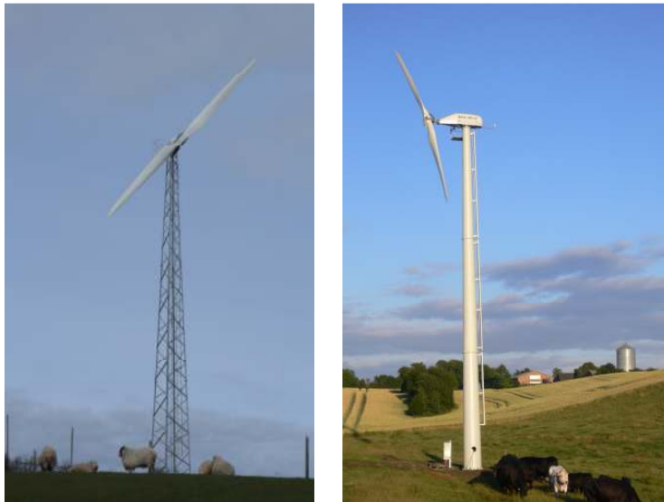
Figure 3.7: Turbine Towers, Lattice (Left) and Tubular (Right)
