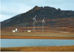
Location — Wales Wind Energy Project, Wales, Alaska Capacity — 0.1 MW Turbine manufacturer — Atlantic Orient Corporation Developer — Kotzebue Electric Association Photo credit — Steve Drouilhet, NREL/PIX09674
