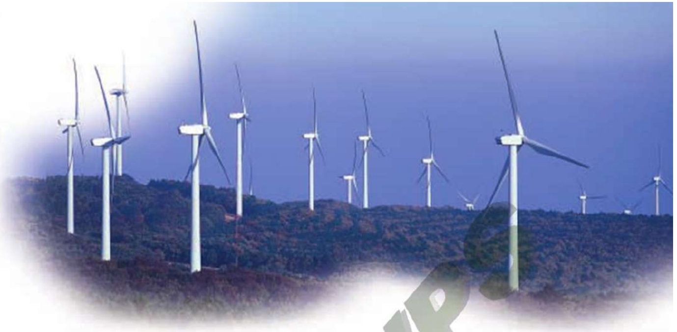
Escurillo, Spain 33 x 1.5sl, total capacity: 49,5 MW
