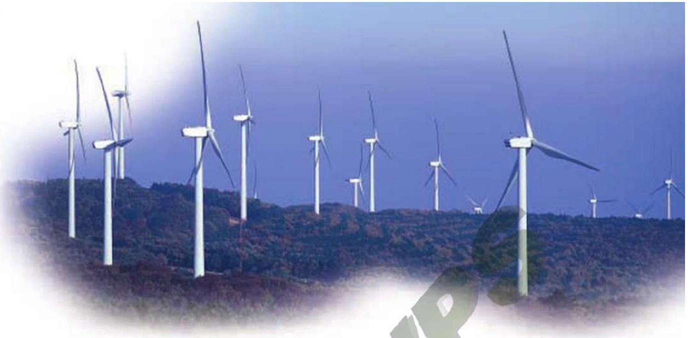
Escorialo, Spain 33 x 1.5sl, total capacity: 49,5 MW
